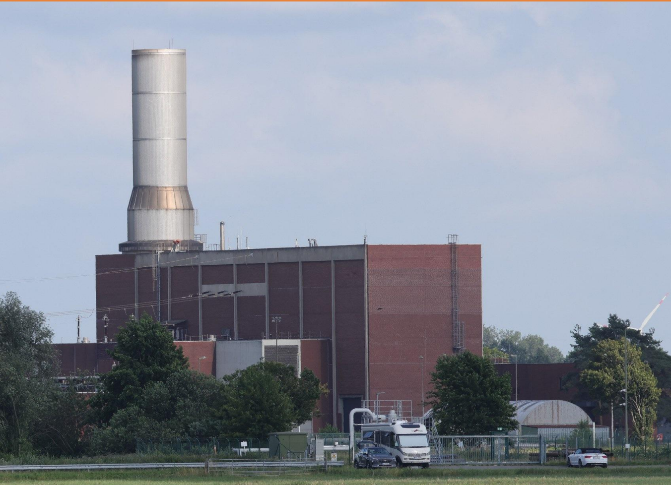
Yingcheng “Energy Storage No.1”: 300 MW / 1500 MWh compressed-air
