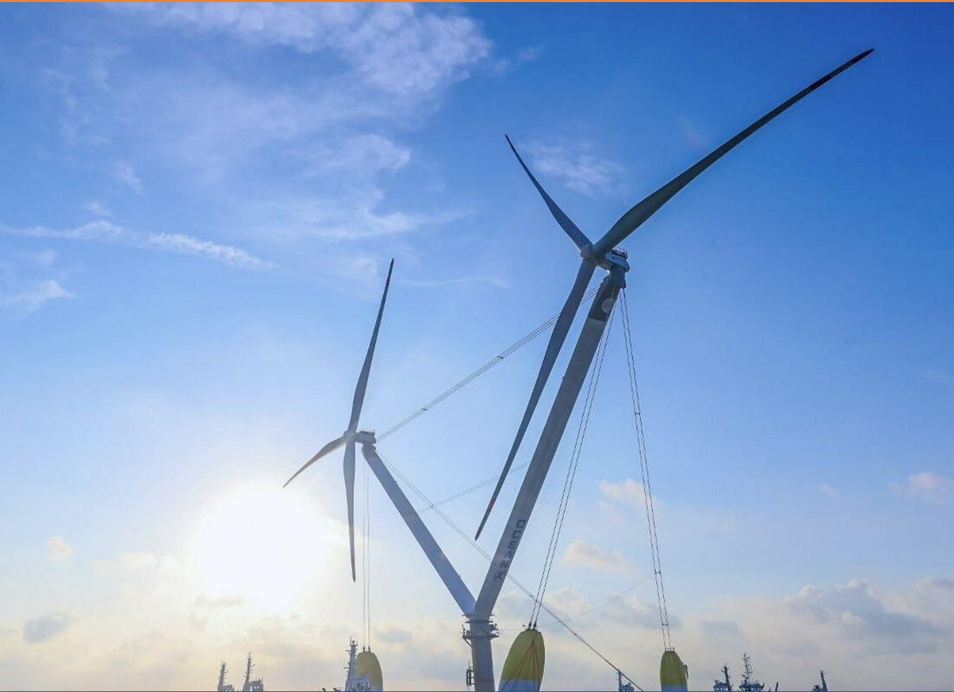
MingYang OceanX: a 16.6 MW twin-rotor floating wind platform
